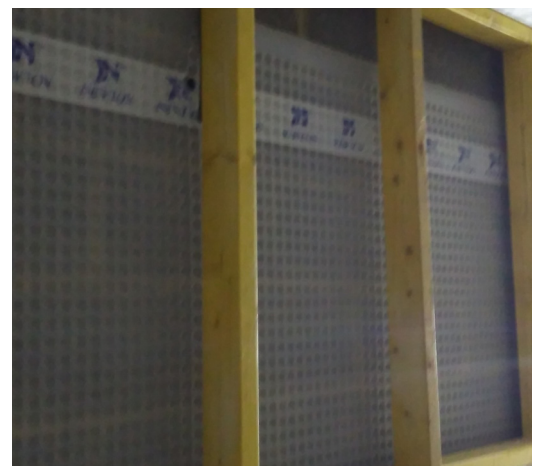
Newton 508 with a new internal timber frame
