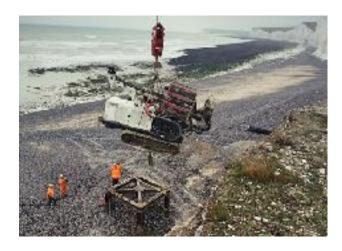
The rig was carefully craned off the cliff down on to the beach and the company carried out bored piling. Once complete, the rig was then craned off the beach and back on to dry land and the steps were then installed The planning of the job was intricate and complex. There were many factors to consider including tidal movements and weather, as the works needed to be carried out in one go in between low and high tide.
