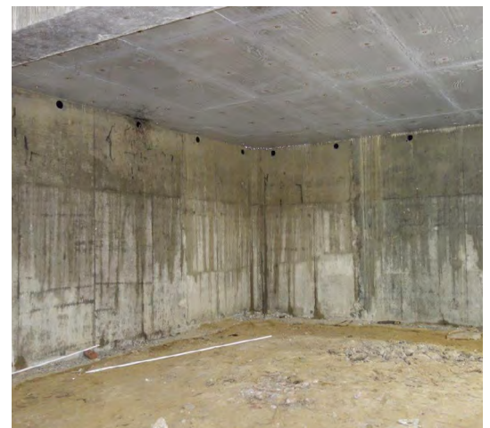
The concrete walls had minor water ingress already
