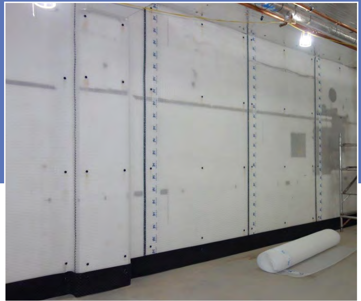
Newton 508 was installed to all of the walls by Advanced Preservations
