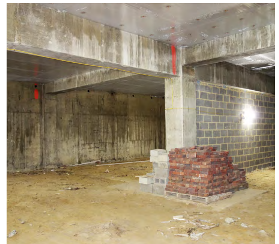
The reinforced concrete walls and internal blockwork
