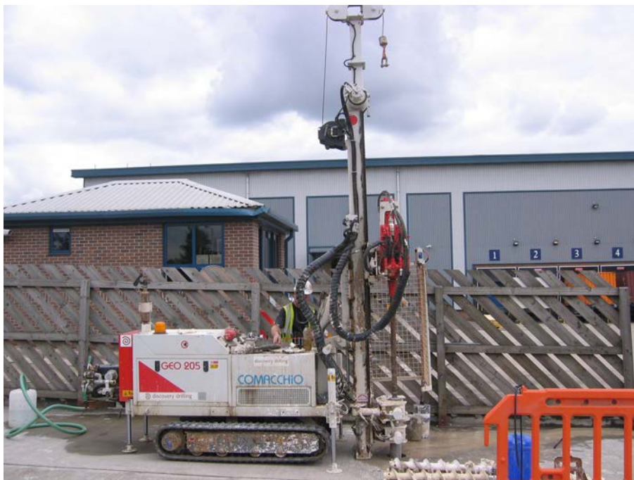
Figure 51. Full access site investigation drilling rig
