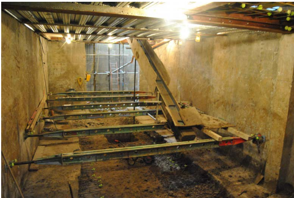
Figure 30. Temporary works - main excavation
