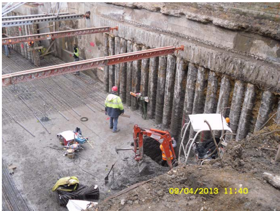
Figure 18. Contiguous bored pile wall
