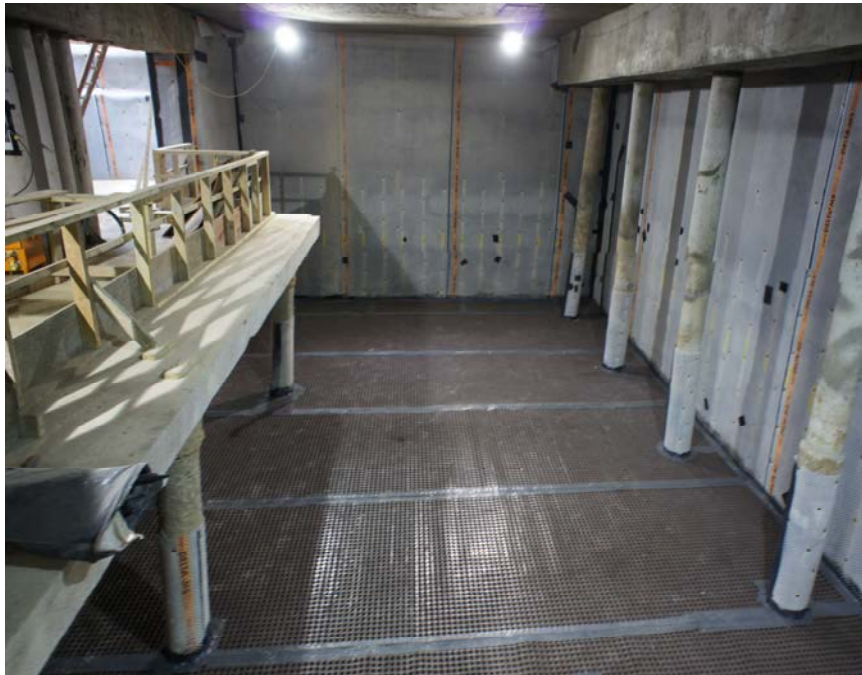
Figure 47. Cavity membrane after installation in a basement
