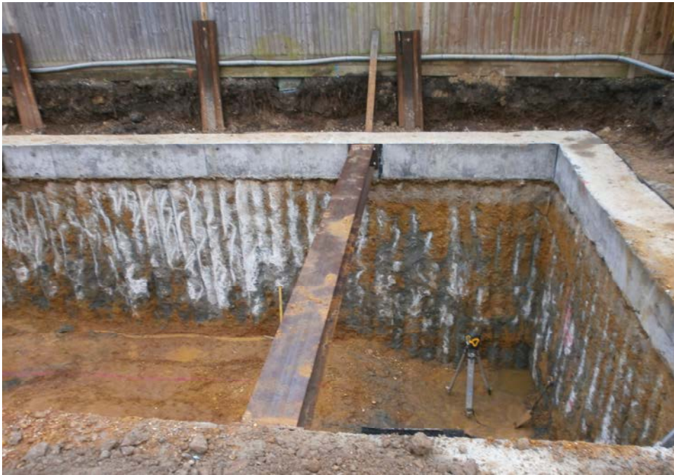
Figure 20. Secant piled wall
