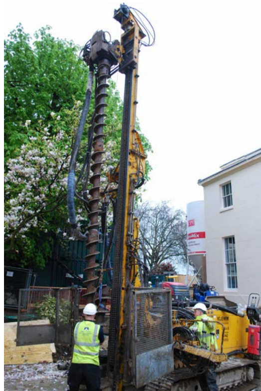
Figure 15. Piling rig in rear garden
