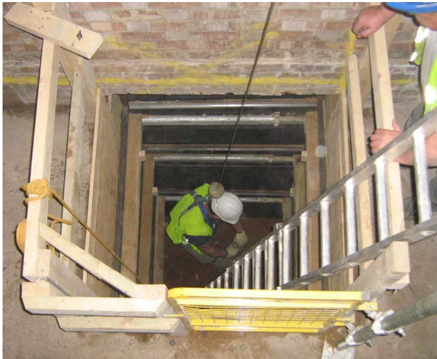
Figure 28. Temporary works - individual underpin
