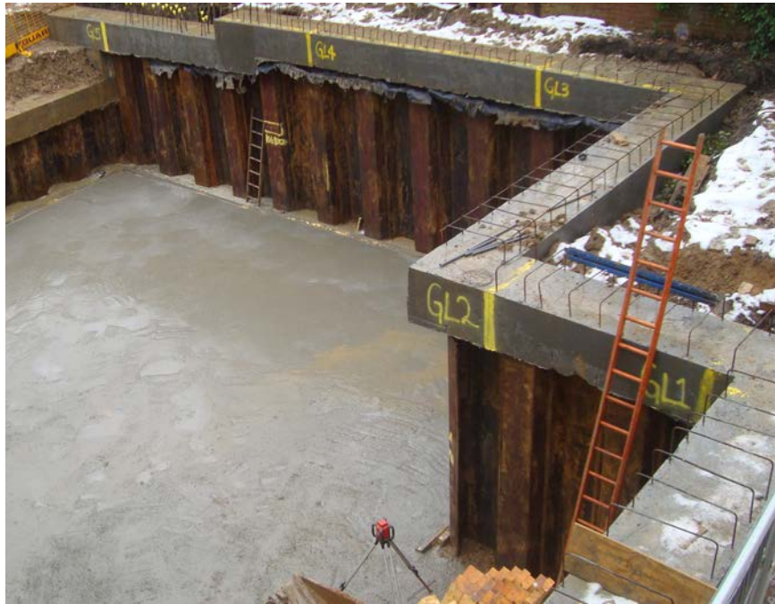
Figure 23. Steel sheet piled wall
