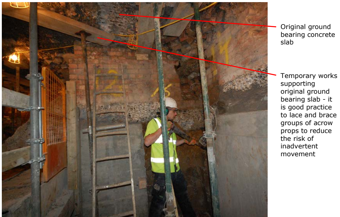
Figure 40. Temporary works during tunnelling below ground bearing concrete slab
