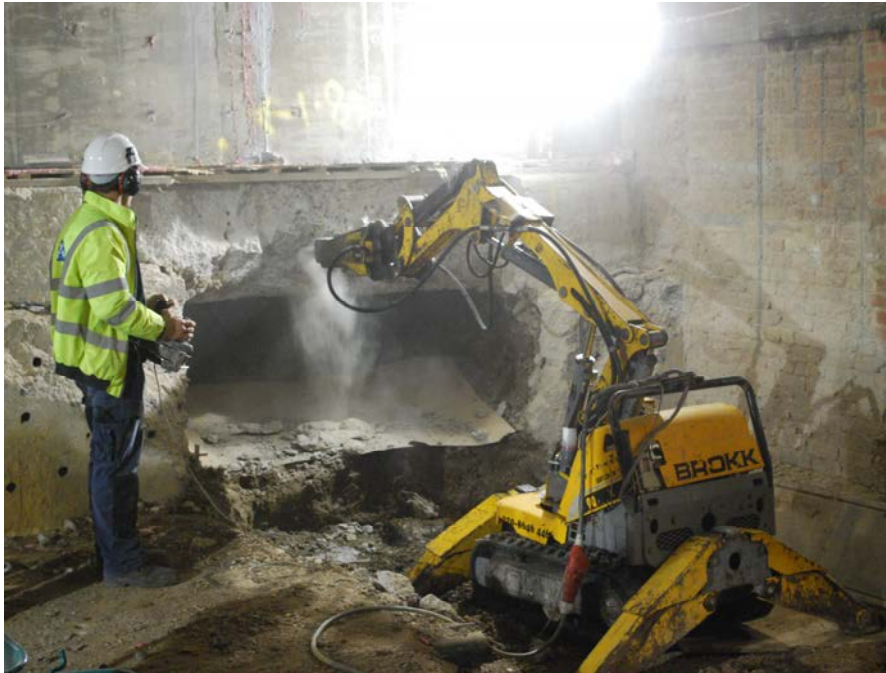
Figure 42. Concrete break out
