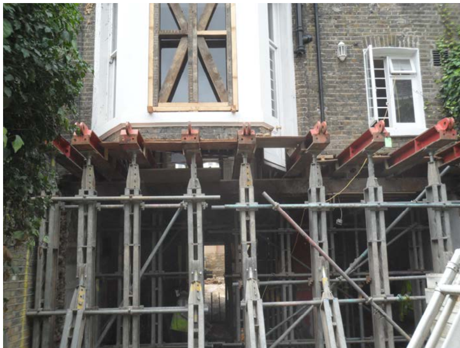
Figure 31. Temporary works - support to existing structure
