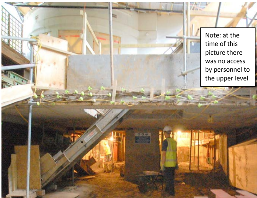
Figure 37. Tunnelling under occupied house
