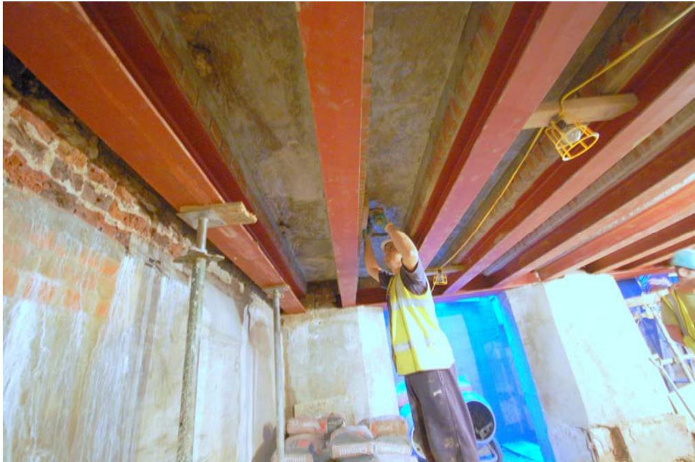
Figure 41. Permanent steelwork to support ground bearing concrete slab
