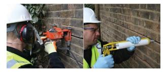
The art of brick reinforcement installation is to create as little disturbance in the brickwork as possible. Often brickwork is old and bedded on weak lime mortars. Standard traditional techniques of brick stitching can cause increased de-bonding in the surrounding brickwork. By using vacuum recovery, low vibration, diamond bladed wall chasers accurate slots to specific set depths in brickwork mortar beds can be made without damaging the bricks.
