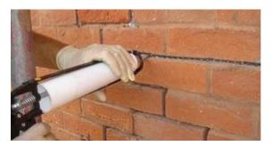
The bed joint can then be re-pointed in colour matched mortar.
