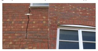
With a toothed chisel carefully out back the mortar along the line of the cracking removing it to a depth of at least 20mm.
