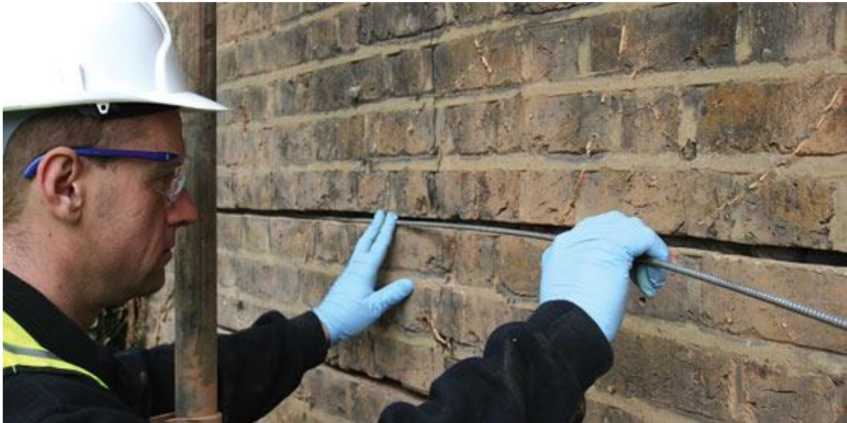
Helical reinforcement being installed in bed joint
