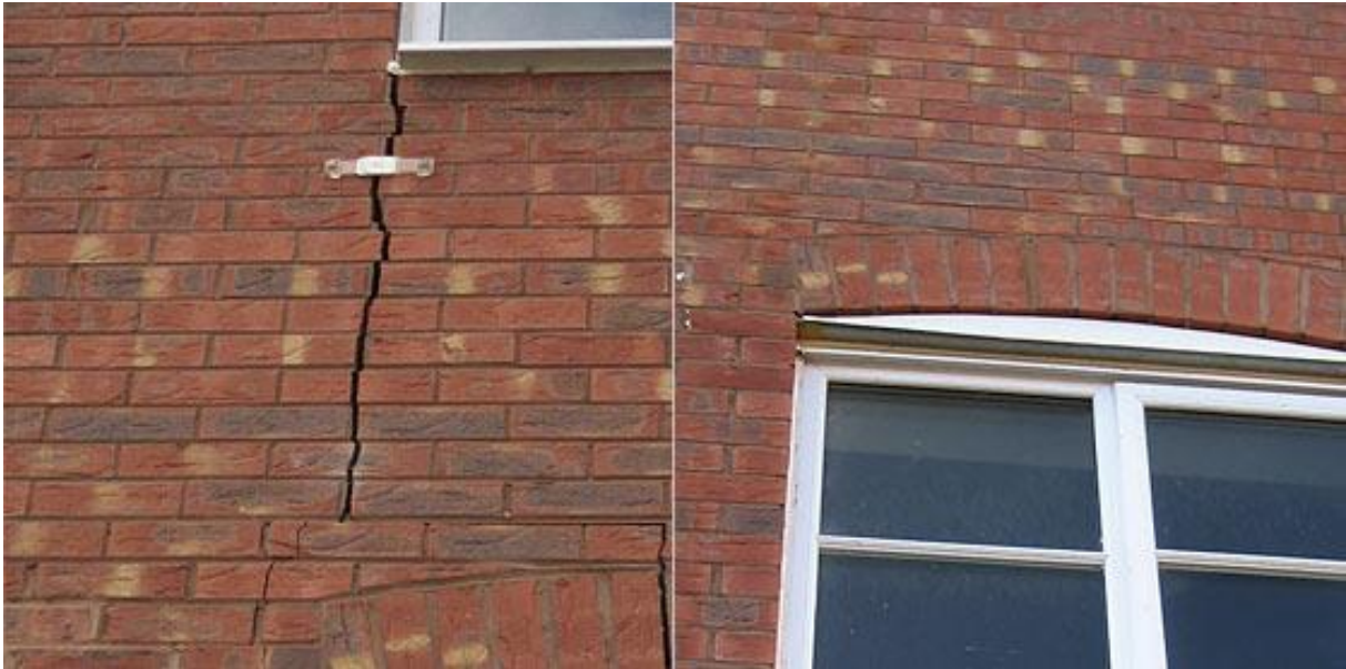
Left: Before work
