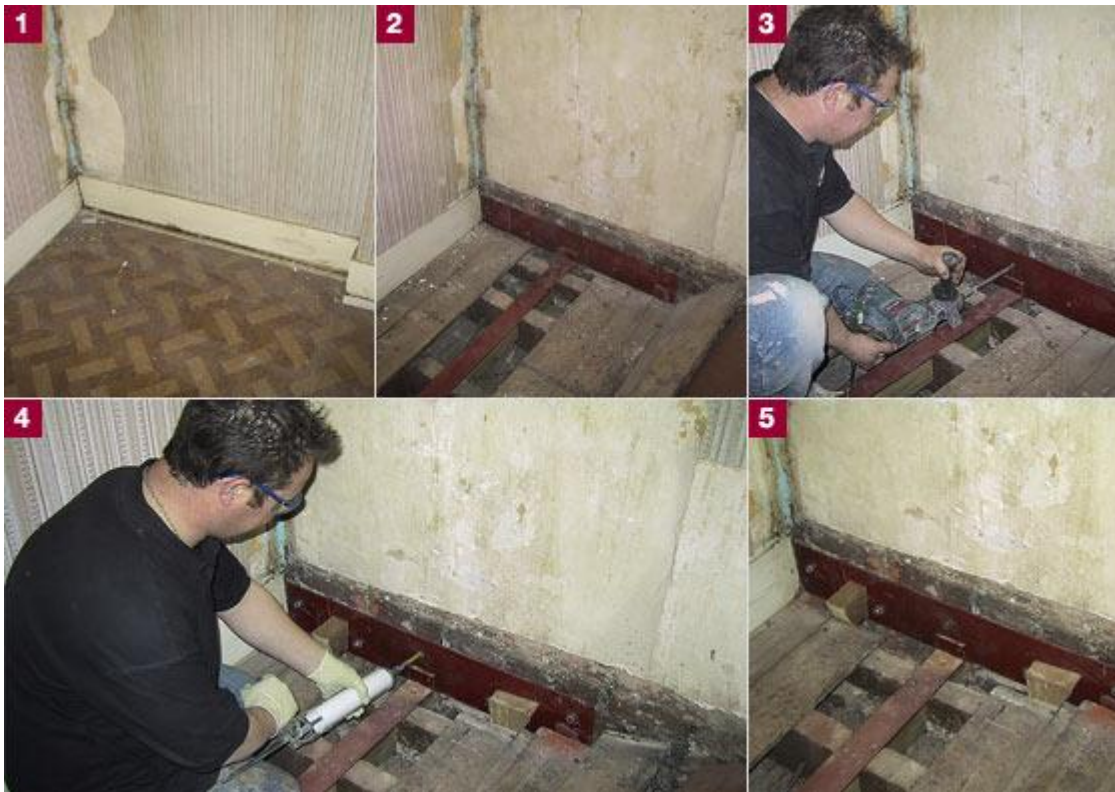
Installation of Tie Bar
