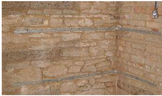
Corner Straps fixed to stone walling with resin anchors
