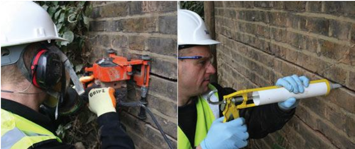
Left: Preparing bed joint using dust-free cutter
