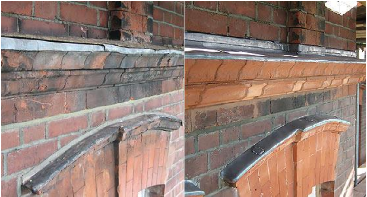
Left: Weathered and aged arch and corbel detail.
