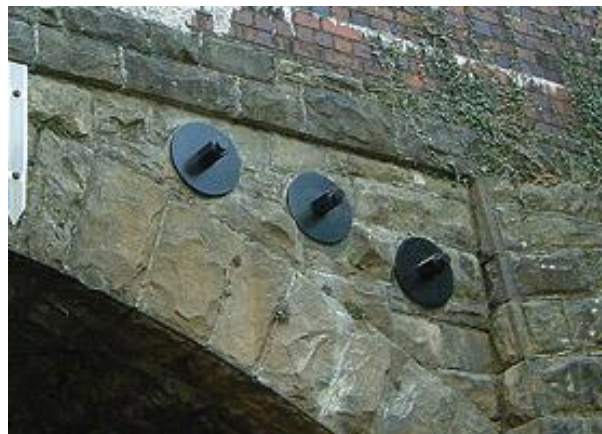
Installed Anchors with Patress Plates
