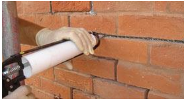
Reinforcement bedded in resin grout
