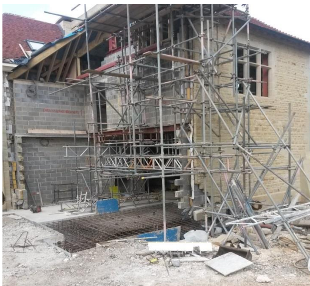
Fig: Temporary works - support to existing structure
