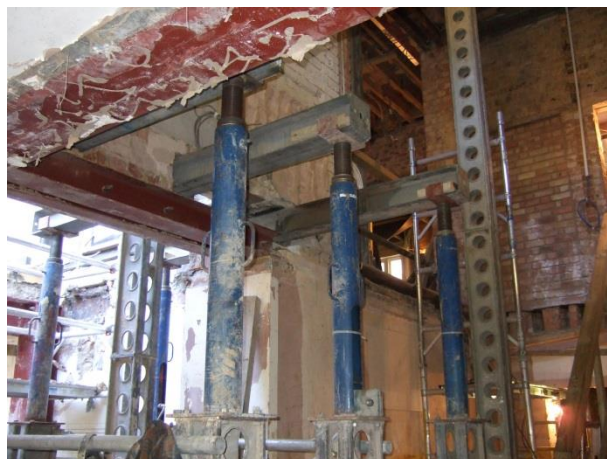
Fig Temporary works - support to existing structure
